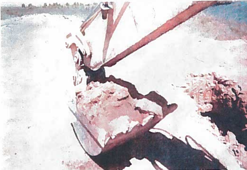
Photograph 14. Bucket the sample from test pit TP-16 was obtained.
