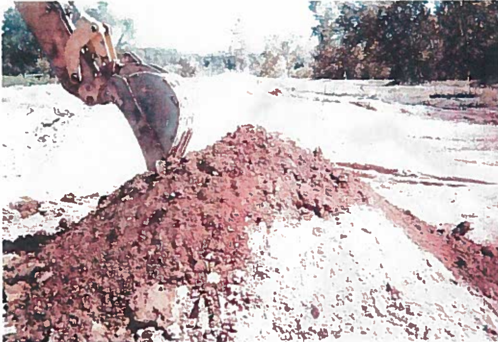
Photograph 21. Spoils from test pit TP-25.
