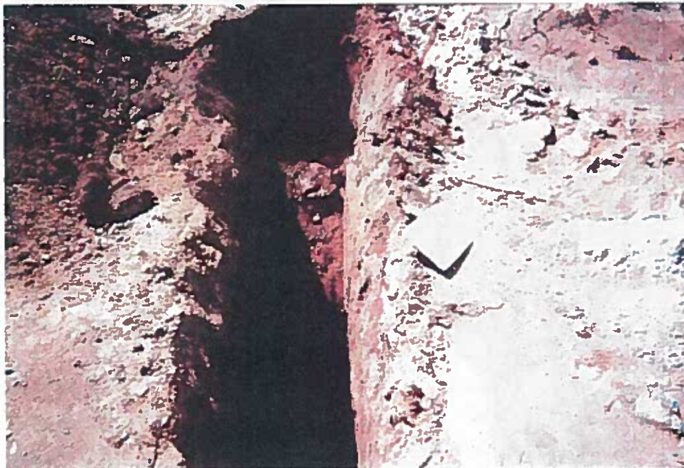
Photograph 22. Test pit TP-27.
