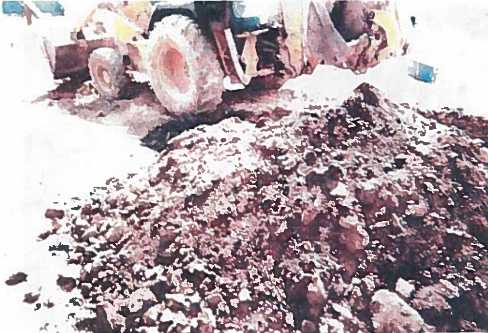
Photograph 5. Spoils from test pit TP-03.
