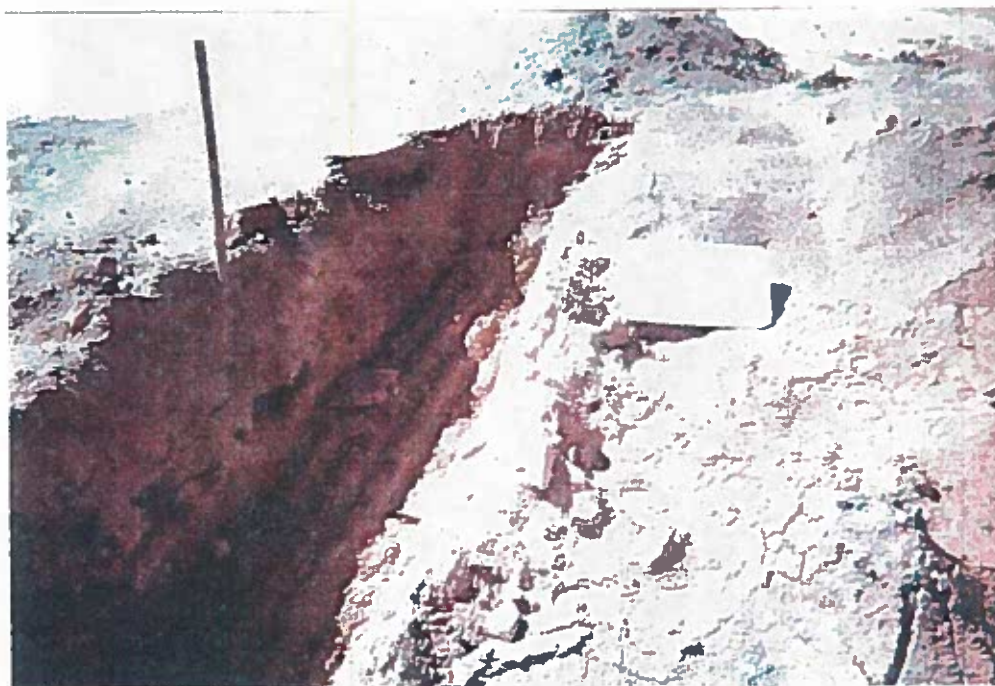
Photograph 20. Test pit TP-25.
