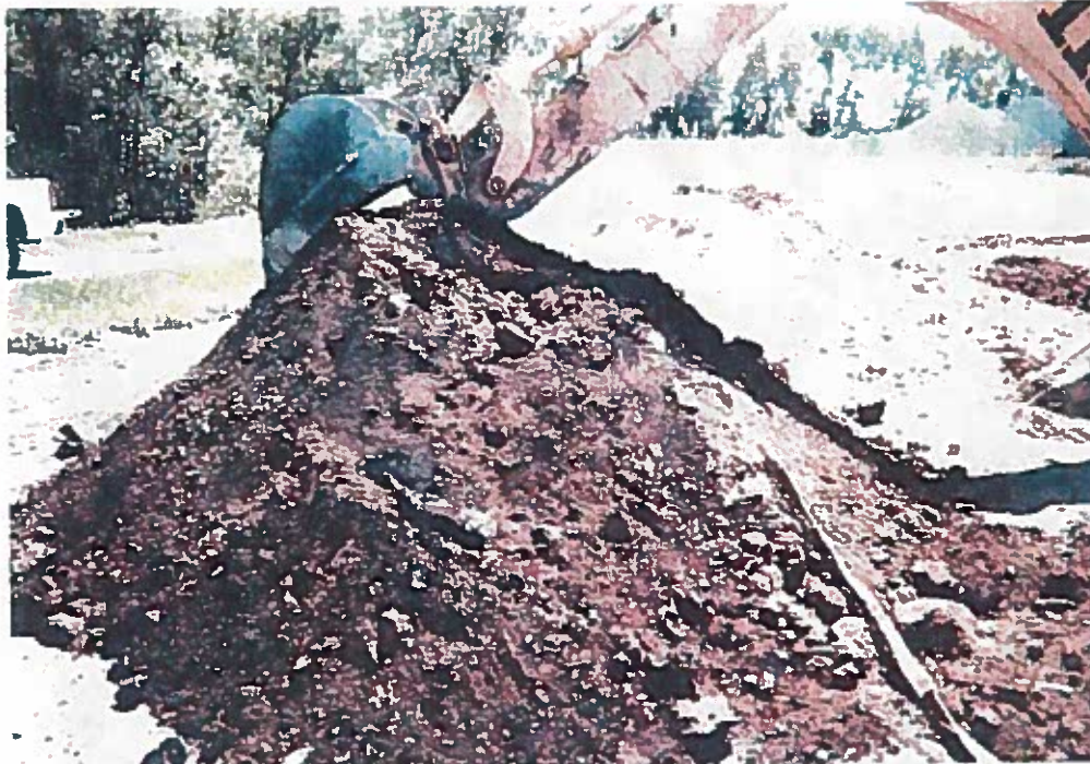
Photograph 15. Spoils from test pit TP-16.
